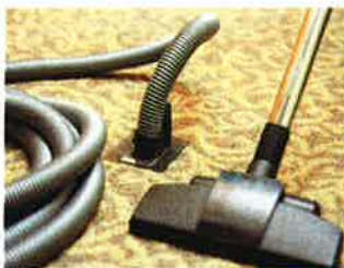
Vacuum Cleaning Inlet
