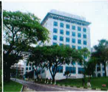
Nanyang Technological University - Technological Plaza Building
