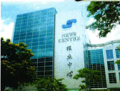
Puzer Clean System for Singapore Press Holdings HQ - 65,000sq.m - 10 floors Highest Tower (Completed 2002)
