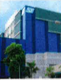
ST Microelectric Wafer Facility - Ang Mo Kio
