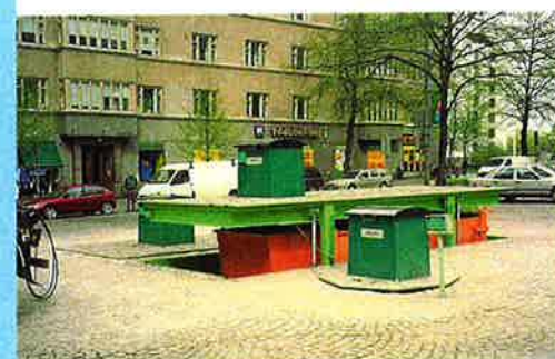
Hidden Refuse Container being raised
