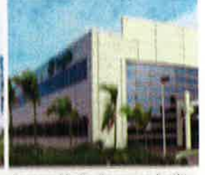
Angsana Malls Operating Facility Woodlands Loop
