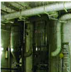
Two-Stage Filtering System Gives Hepa Quality discharge air meeting PM2.5 - Air Quality Standard.
