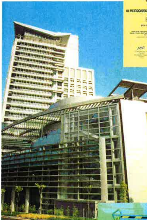
Puzer Protect System Installed for 30floors (60,000 sq.m) Ministry of Education HQ Building for Waste Paper Recovery Integrated with Central Vacuum Cleaning (Completed 2000)
