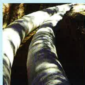
buried refuse pipes
