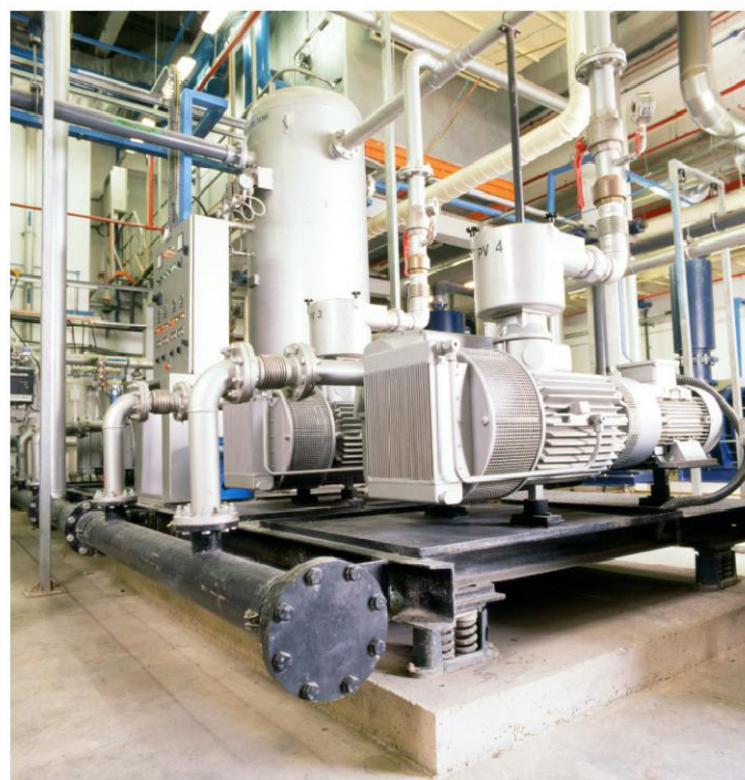
4 x 600 Actual m 3 /h Oil Lubricated Vacuum Pump Package
