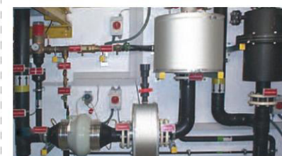
Exhaust air filter system for decay tanks
