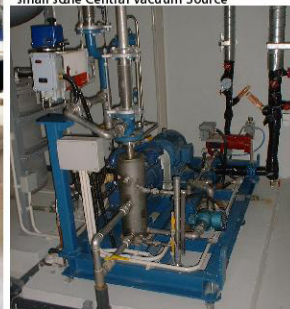
Three Stage Oil Free Vacuum Pump Package For Life Science Research
