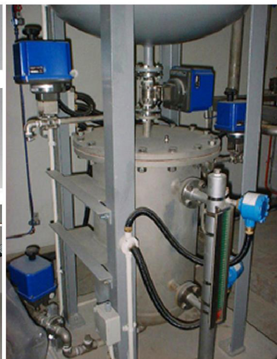
Moisture Extracting System with PH Monitoring for Life Science Research Facility
